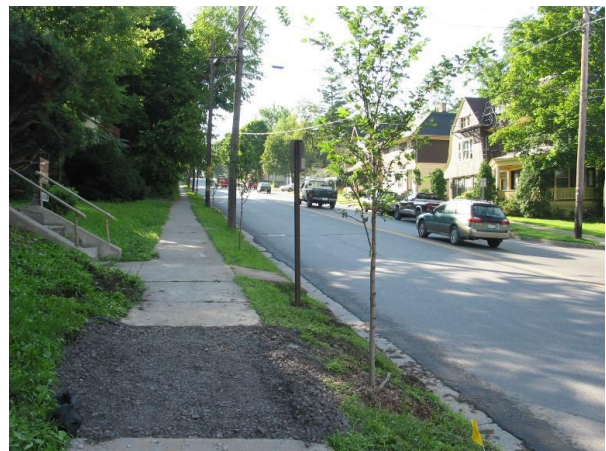
Because this tree lawn is so narrow, a sidewalk section has been removed, and a replacement will be poured on this CU- Soil® base. Ithaca, NY
