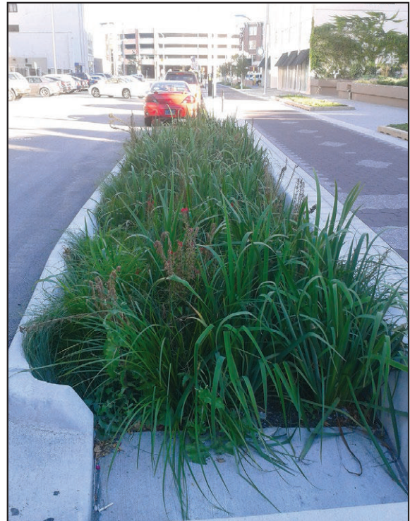
Examples of bioswales in downtown Indianapolis, IN. Left bioswale is in need of maintenance and revegetation; right bioswale is well vegetated and appears to be working properly.
