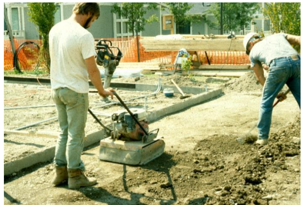
Compaction of soil in preparation for pavement
