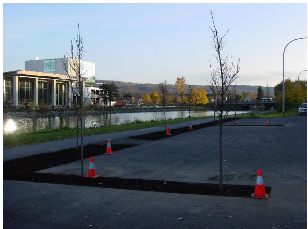
The finished parking lot
