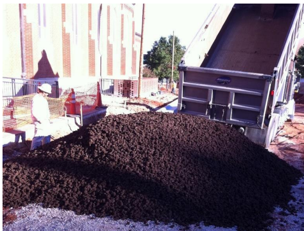
CU-Structural Soil® being delivered to project site. Photo courtesy Minick Materials Company
