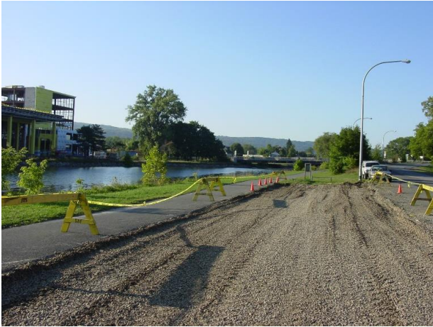
CU Structural Soil® was used as a 2' deep base course for the entire parking lot
