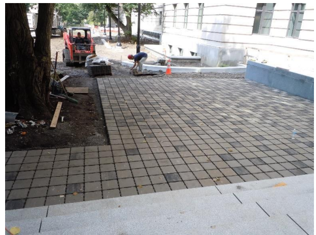
Permeable pavers were installed over the CU-Soil® and mature tree roots
