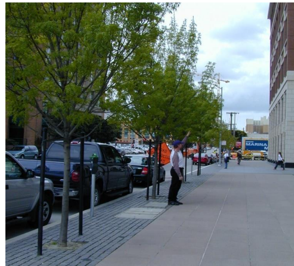
This installation uses cobble pavers with porous joints as the covering of a continuous trench of CU-Soil®.
