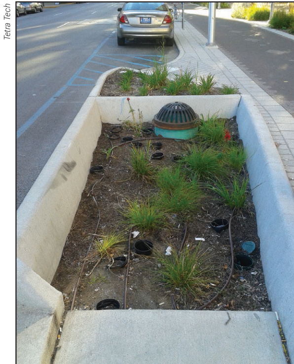
Examples of bioswales in downtown Indianapolis, IN. Left bioswale is in need of maintenance and revegetation; right bioswale is well vegetated and appears to be working properly.
