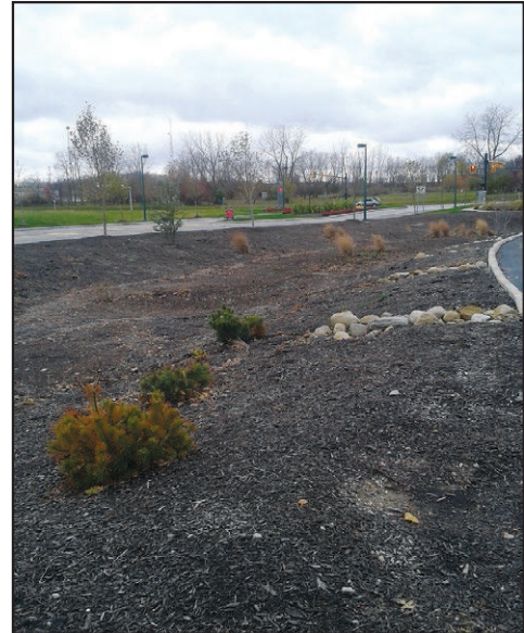
Lack of vegetation in bioretention area (Beachwood, OH)
