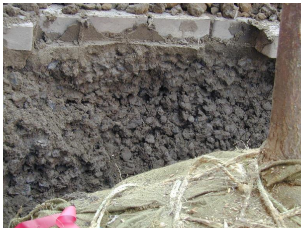
Closeup of CU-Structural Soil® after installation
