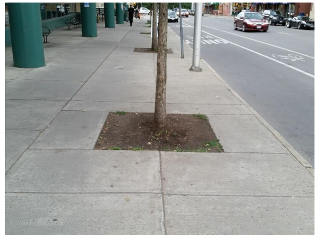
A continuous trench of CU-Soil® connects each tree pit to one another
