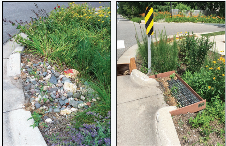
Figure 1. Two types of street raingarden inlets: Left – Rock inlet; Right – Pretreatment inlet. The pretreatment inlet is now required for all new street raingardens to aid in collection of gross solids (sediment, leaves, trash, etc.) and maintenance. Rock inlets are no longer allowed due to difficulty maintaining the effectiveness of the inlet for pretreatment.
