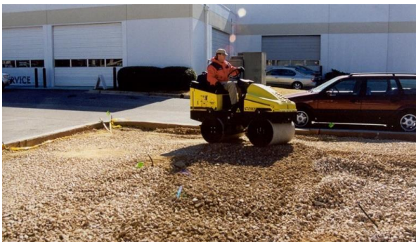
Compaction of CU-Structural Soil® prior to installing sod. Photo courtesy Southpine, Inc.
