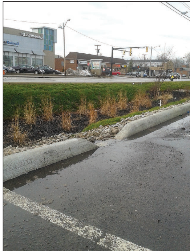
Bioswale treating runoff from urban parking lot (Cleveland, OH).
