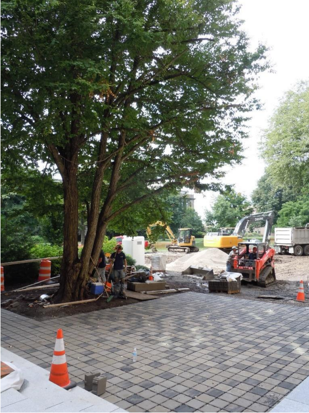
The nearly finished plaza space
