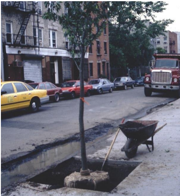
The standard (but entirely inadequate) city tree pit. It's not surprising that trees in these situations have shorter lifespans.
