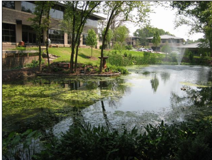
Photograph WQ-2 – Example of an Extended Wet Detention Basin.
