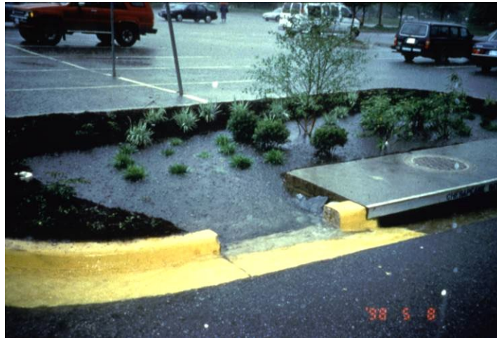
Photograph WQ-4 – Example of Porous Landscape Detention.
