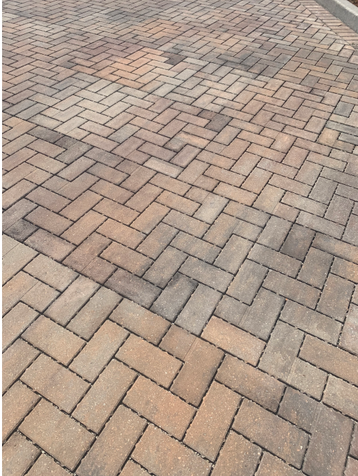
Photograph WQ-7 – A variety of designs are available for porous pavement that can be selected to best fit the site surroundings.
