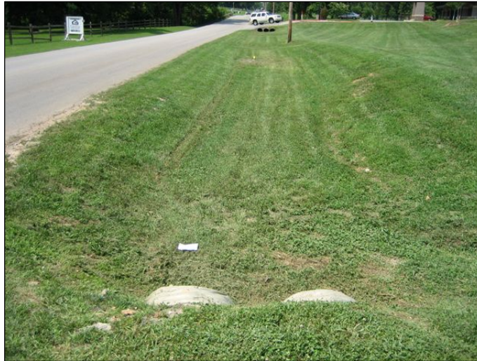
Photograph WQ-9 – Example of a Grass Swale.
