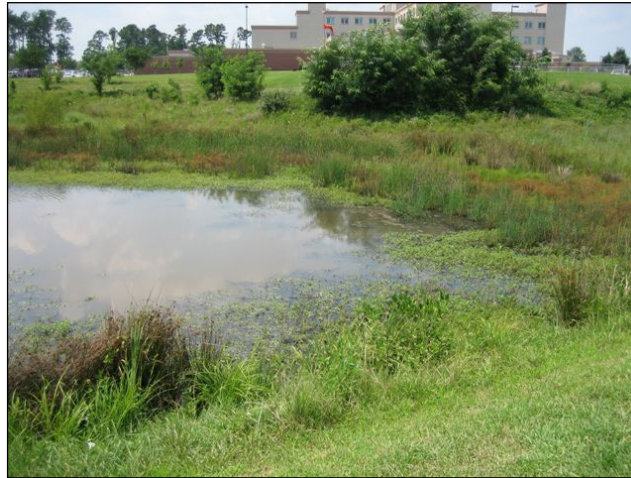
Photograph WQ-3 – Example of a Constructed Wetland Basin.
