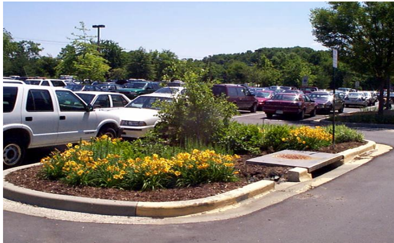
Photograph WQ-13 – Example of a Porous Detention Island. This porous detention island is designed to reduce runoff rates and volumes and pollutant loading.
