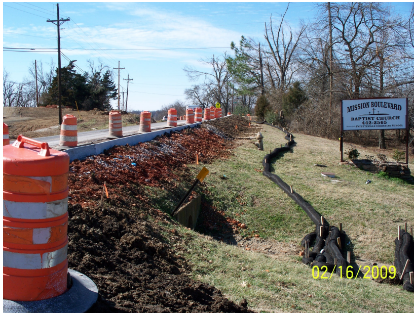
Photograph CS-7 – Example of Fiber Roll/Wattle
