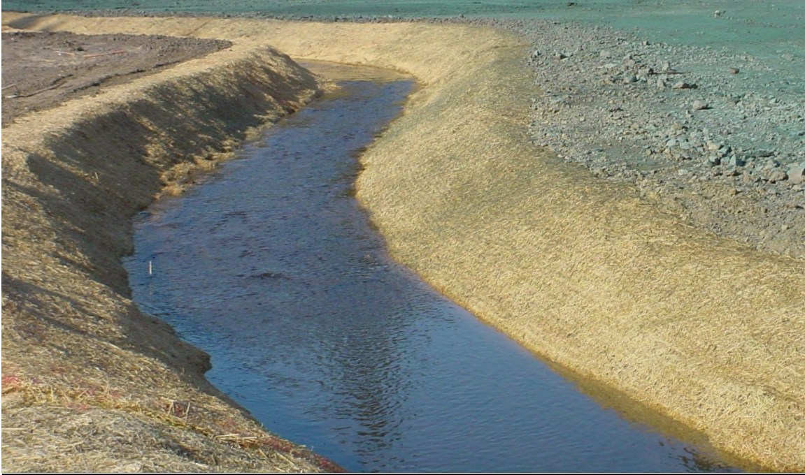
Photograph CS-3 – Example of Erosion Control Blanket
